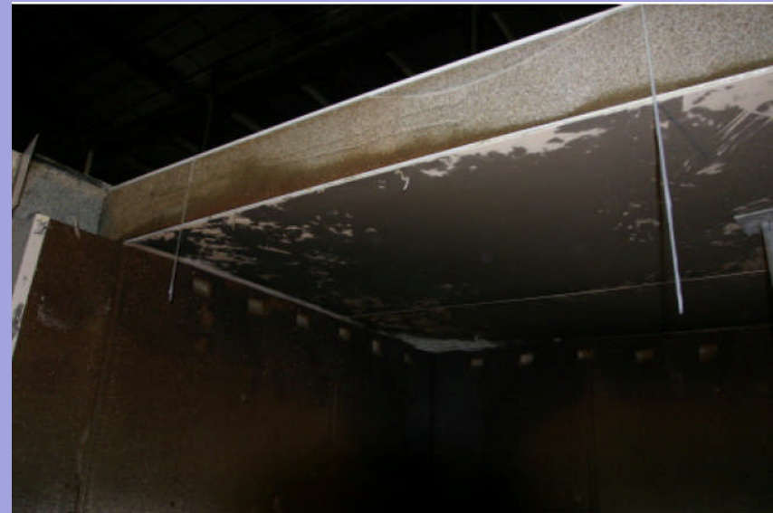
Figure 10. Depth of char/discolouration in ceiling panel 8.
